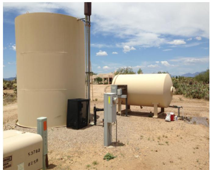
Figure 1. Shared Well storage and pressure tanks. Source: G. Hix.
