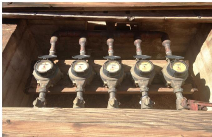
Figure 2. Shared well metered service connections with shutoff valves. Source: G. Hix.
